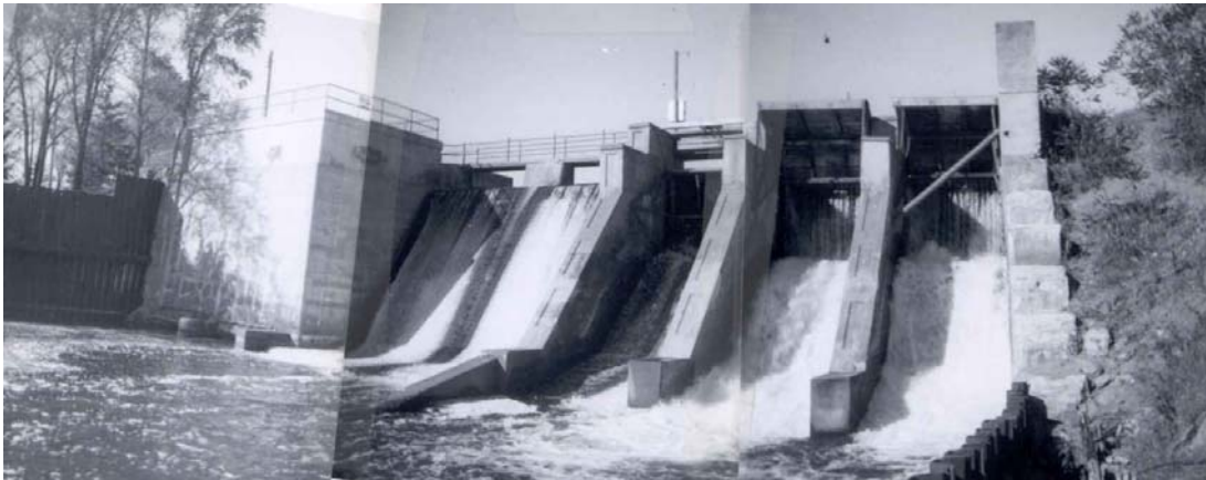
Figure 10. The Black Brook Dam
